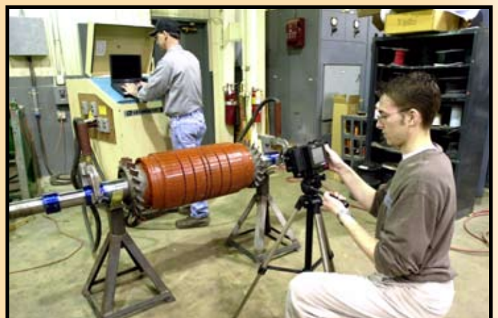
An infrared camera is used to determine hot areas on rotors and stators.
